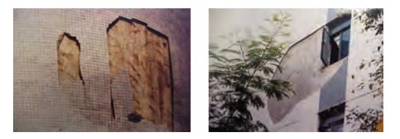
Concrete buildings in Hong Kong, though impressive, suffer from the same problems experienced by concrete the world over. That is, they contain steel reinforcement, which readily rusts in the humid atmosphere that prevails here through most of the year. In addition, the surfaces of many buildings are rendered over and some are also tiled. Joints to allow for movement are seldom incorporated in the surface and as a consequence often pieces fall off. Maybe they should be fibre reinforced!
